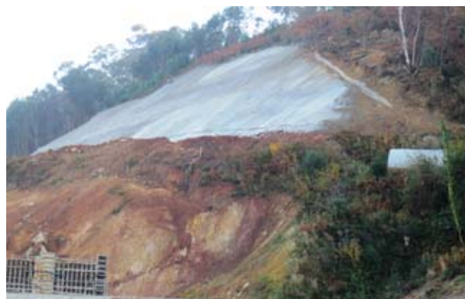
Figure 7. Slope picture after placing soil-nailing in the top half.
